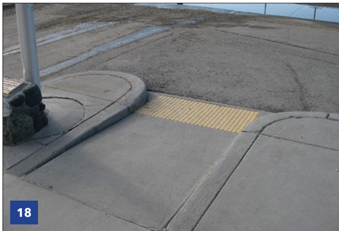
18 Ramped curb cut with truncated domes.
